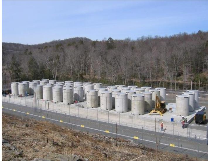
Figure 19.4.2-7: Typical layout of dry cask storage site. [19-39]
